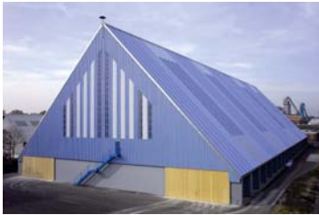
Road salt building
