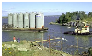
Floating silos in the fjords, Norway
